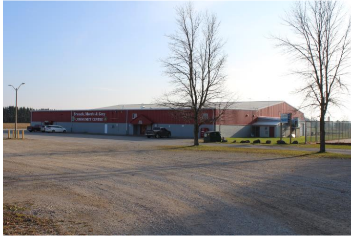
BMG Arena/Community Centre
