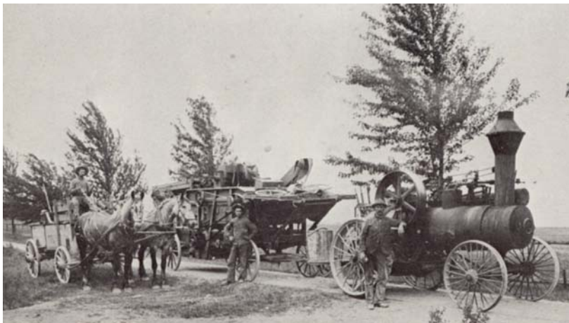
Robert Bell and John Finlayson bought Coleman's Foundry in 1899. The Robert Bell Engine & Thresher Co. was formed in 1903 and, in 1905, the first threshing separator was made. A threshing outfit and the foundry buildings are pictured in the photographs.
