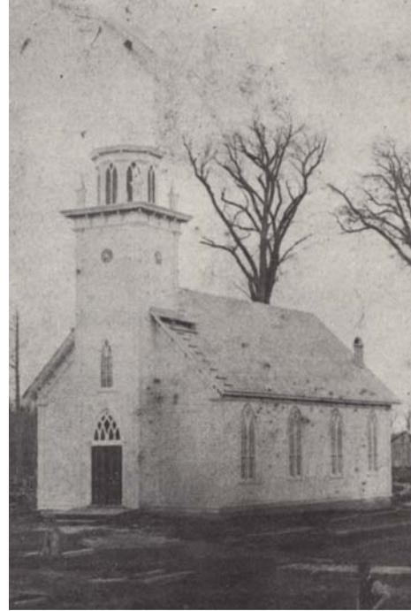
Building the Church in 1863 Photo: Public Archives of Canada
