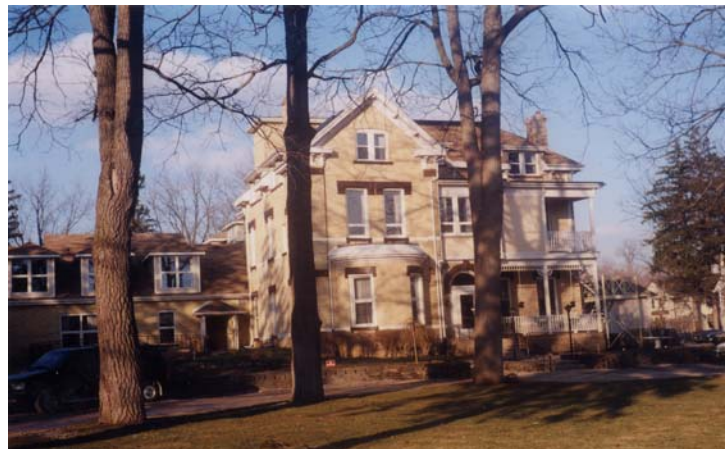
Note the dark window labels and sills accentuating each window and door opening, as well as the decorative cornice brackets.
