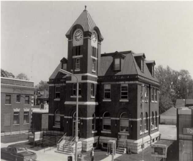
Note the rusticated stone foundation and the use of the white stone in the banding
