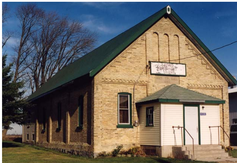
The date stone reads: Grey Tp. Hall 1892. Note the raised decorative brickwork of the gable end and the pilasters marking the corners and bays.
