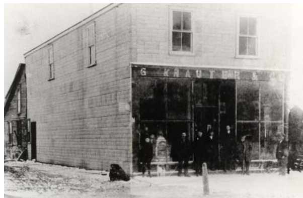
The George Krauter hardware and tinware store plus broom factory, c. 1906.
