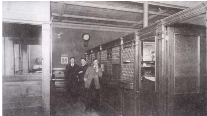
The interior of the bank showing the decorative, and protective, cast-iron tellers' cages.
