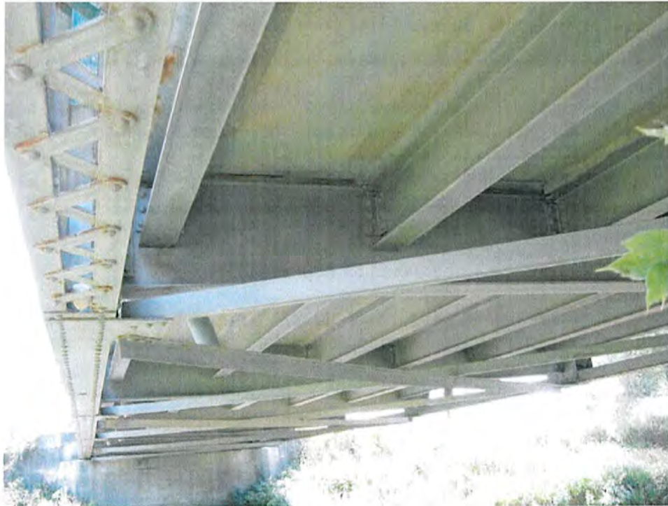
T13 – Kinburn Line – Soffit
