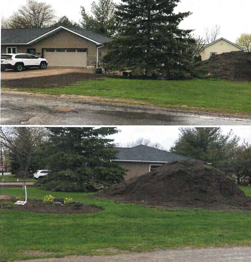
Figures 5 & 6: Image of existing house and approximate location of proposed shed
