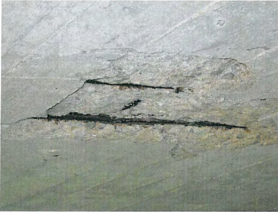
M10 – Hensall Road – Delamination and spalling
