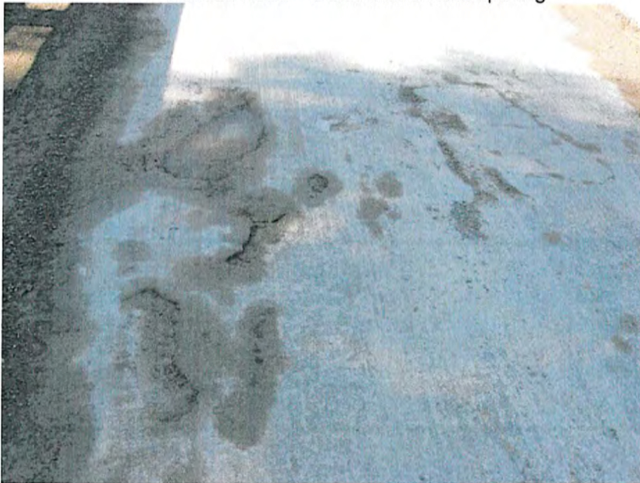
M10 – Hensall Road – Delamination and spalling
