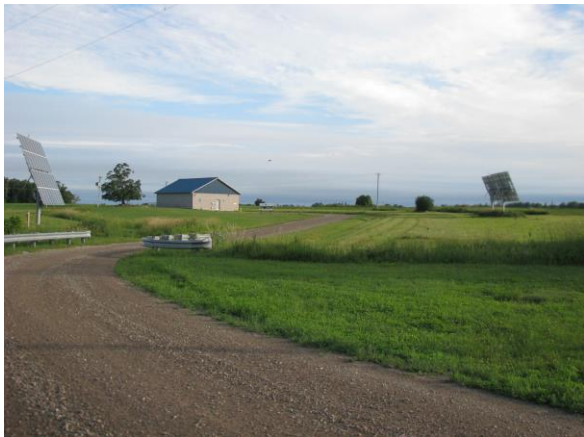
10 kw Solar Trackers at Seaforth Water Plant
